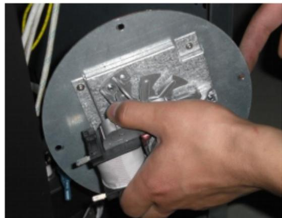
Figure 28: Combustion Motor Assembly
